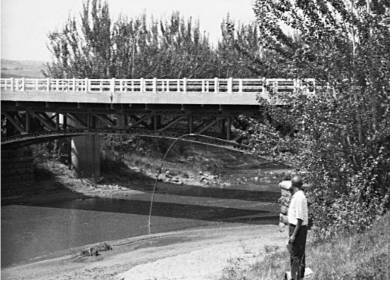
Original method of extraction: small pipe from bridge into river (in centre of picture), with local WASA officer
