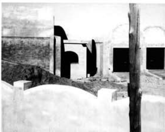
House under construction, Verwoerdburg. 22 June 1986.
