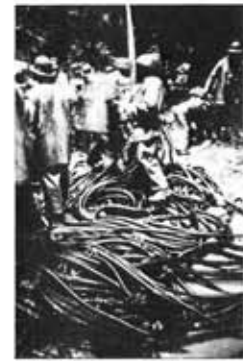
59. Shaft sinking: connecting hoses for drilling. President Steyn No. 4, Welkom. 1969 (E9019)
