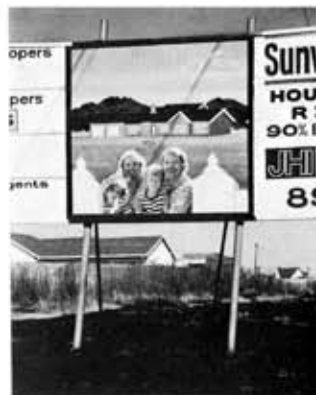
183. Property developers' billboard, Sunward Park. May, 1980 (4-2684)
