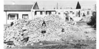
154. Salvaging bricks from demolished houses. 3 June, 1982 (4/2879)
