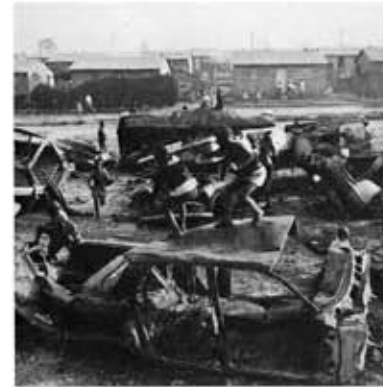
80. Playground, Soweto. September, 1970 (2/11403)
