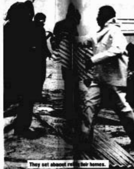
They set about rebuilding their homes.
