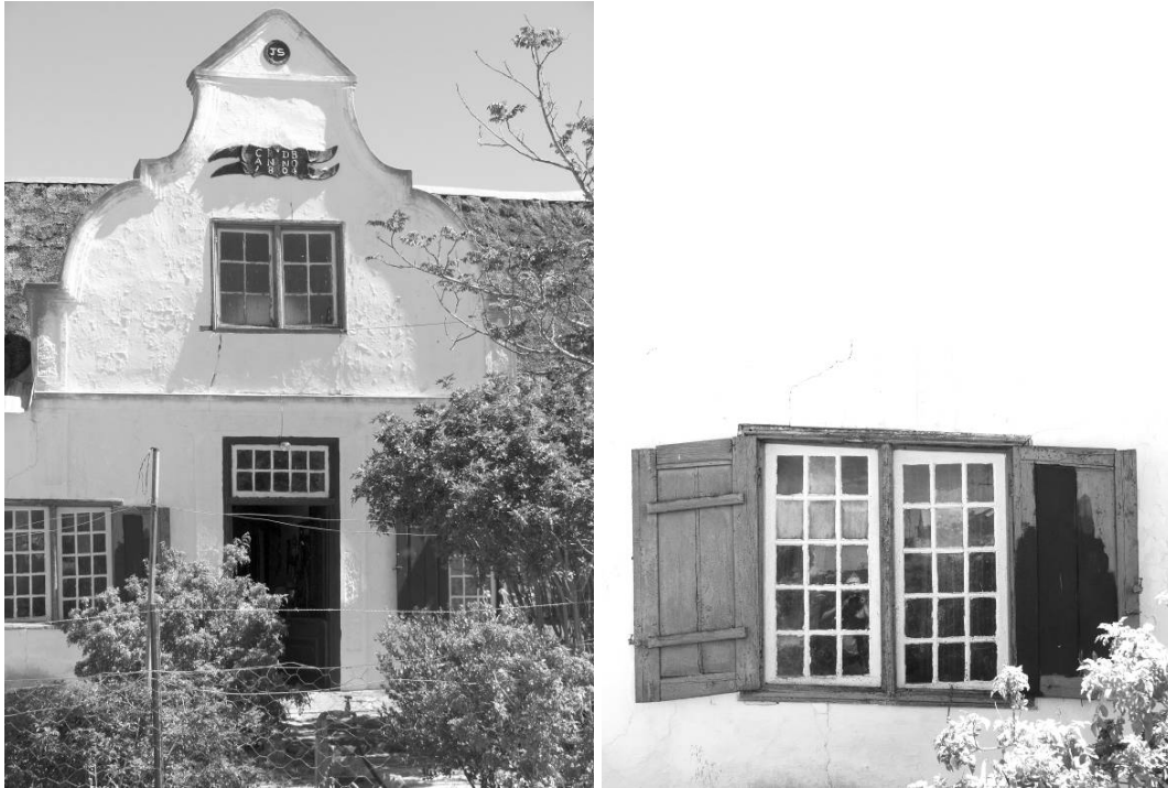
Figure 3. The front gable and detail of casement window.
