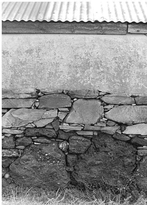
Figure 5: Wall construction of house at Melkhoutrivier near Infanta showing that at the base of the wall the heaviest stones were used (photo EB 1992).
