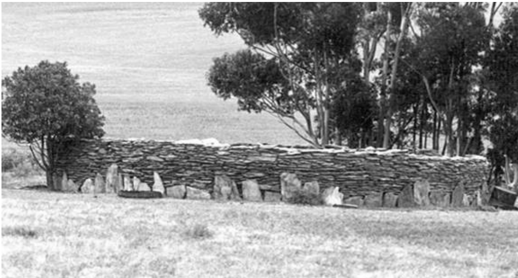
Figure 1: Wall construction: Tarentaalsrivier stone kraal (photo EB 1992).
