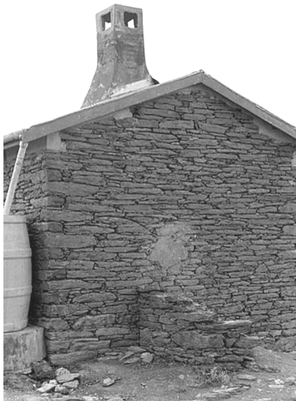
Figure 3: Kraaiheuvel house showing the use of large stones on the corners of the walls (photo EB 1991).
