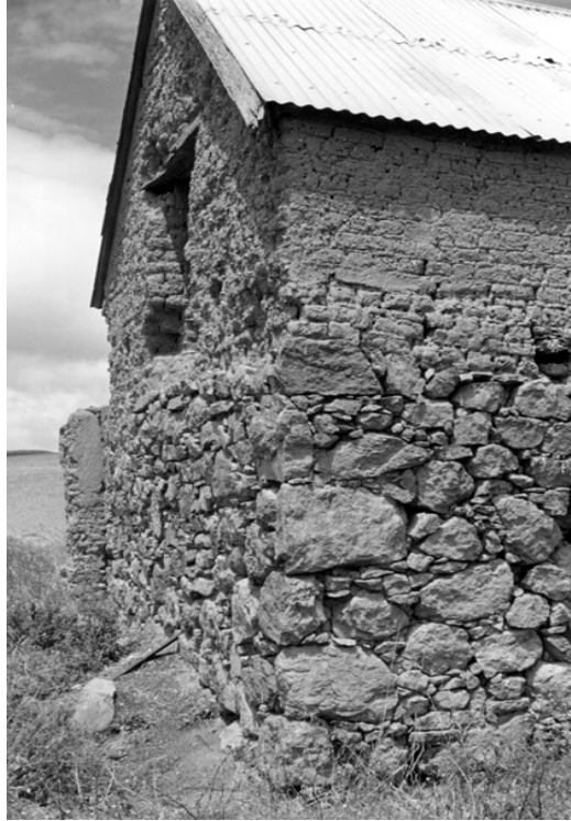
Figure 4: Klaaskaffersheuwel longhouse showing the use of sandstone (koffieklip) (photo EB 1992).
