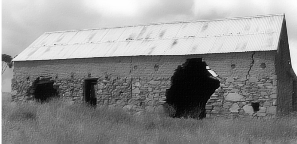
Figure 15: North view of Klaaskaffersheuwel longhouse, with the living quarters to the east and the stable to the west built in two stages – note the use of different stone and the level of the ends of poles (photo EB 1992).
