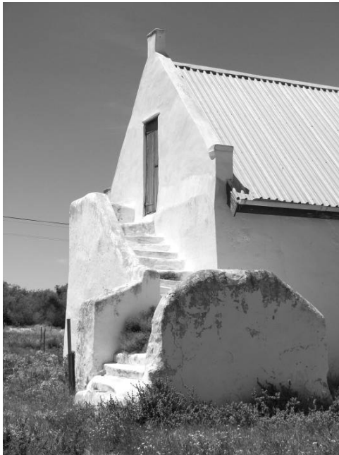
Figure 6. Original thatch is replaced with corrugated iron, and the outbuildings are stabilized.
