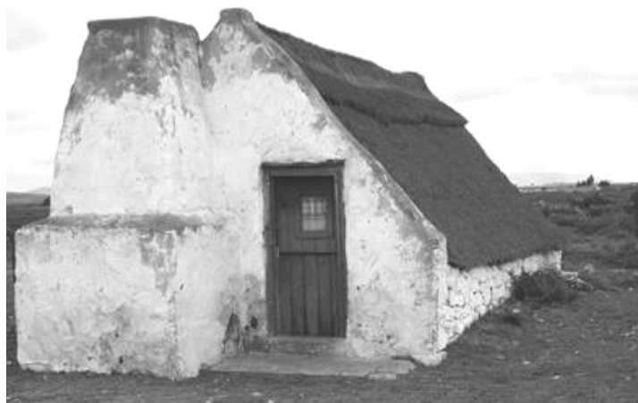
Figure 13: Duinerug, end gable with chimney attached outside (photo EB 1992)
