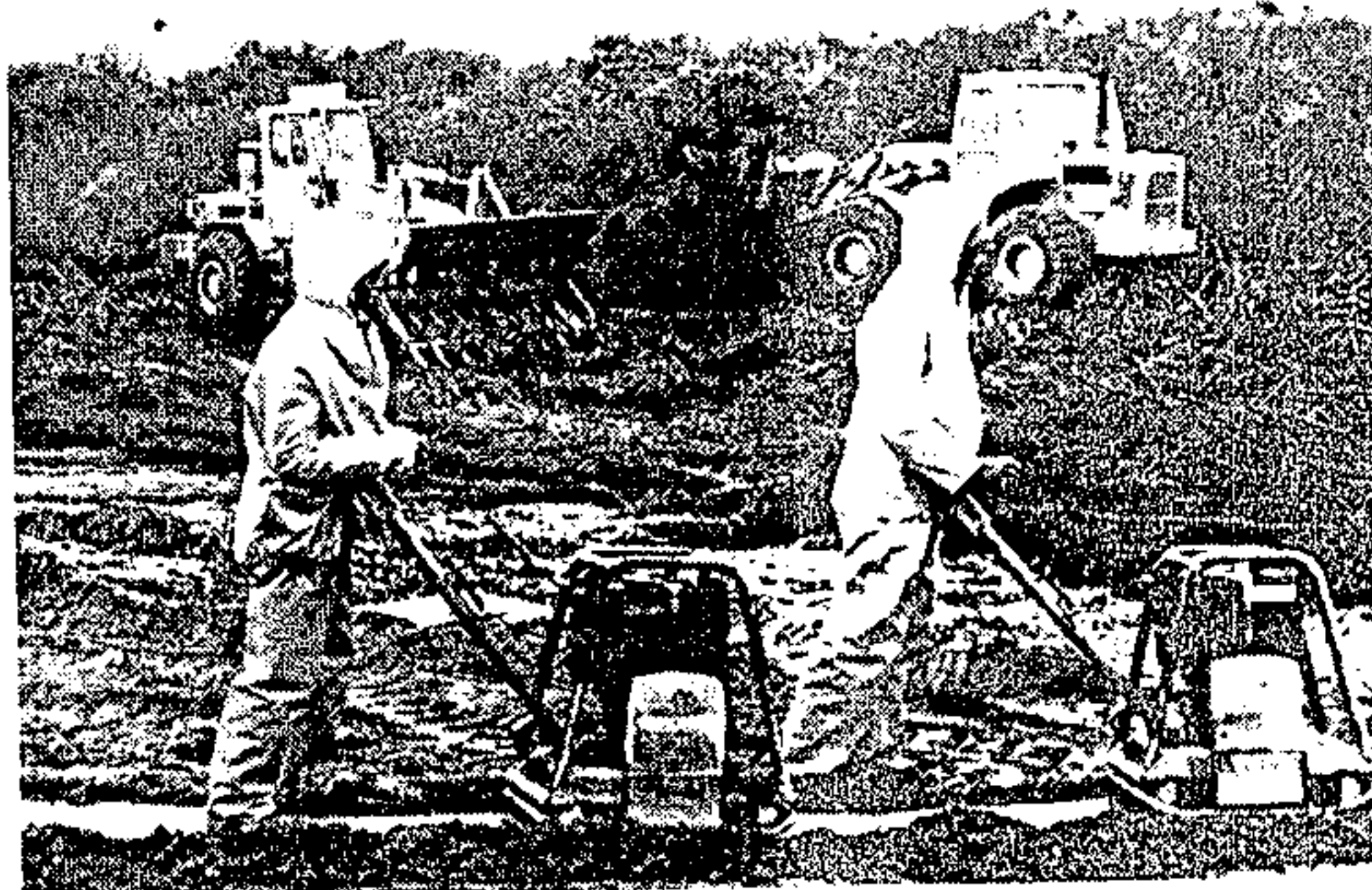
CLEARING THE LAND . . . and levelling it, to make way for houses on Blue Downs. Work has already started on the relatively up-market development.
