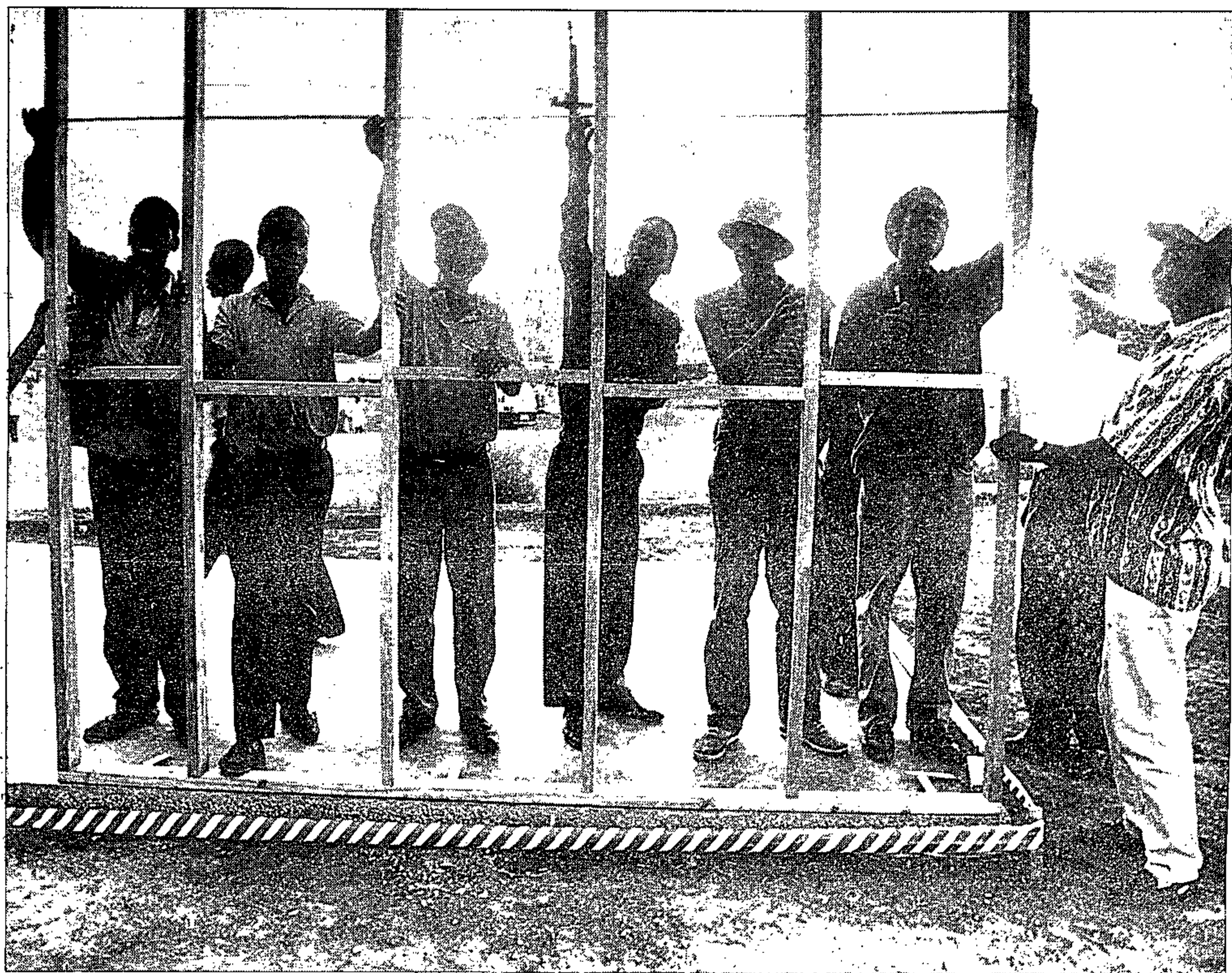
Shaky foundations ... reconstruction was part of the promised packages, but there have been mixed feelings about whether this, or the Masakhane Campaign, has got off the ground.
