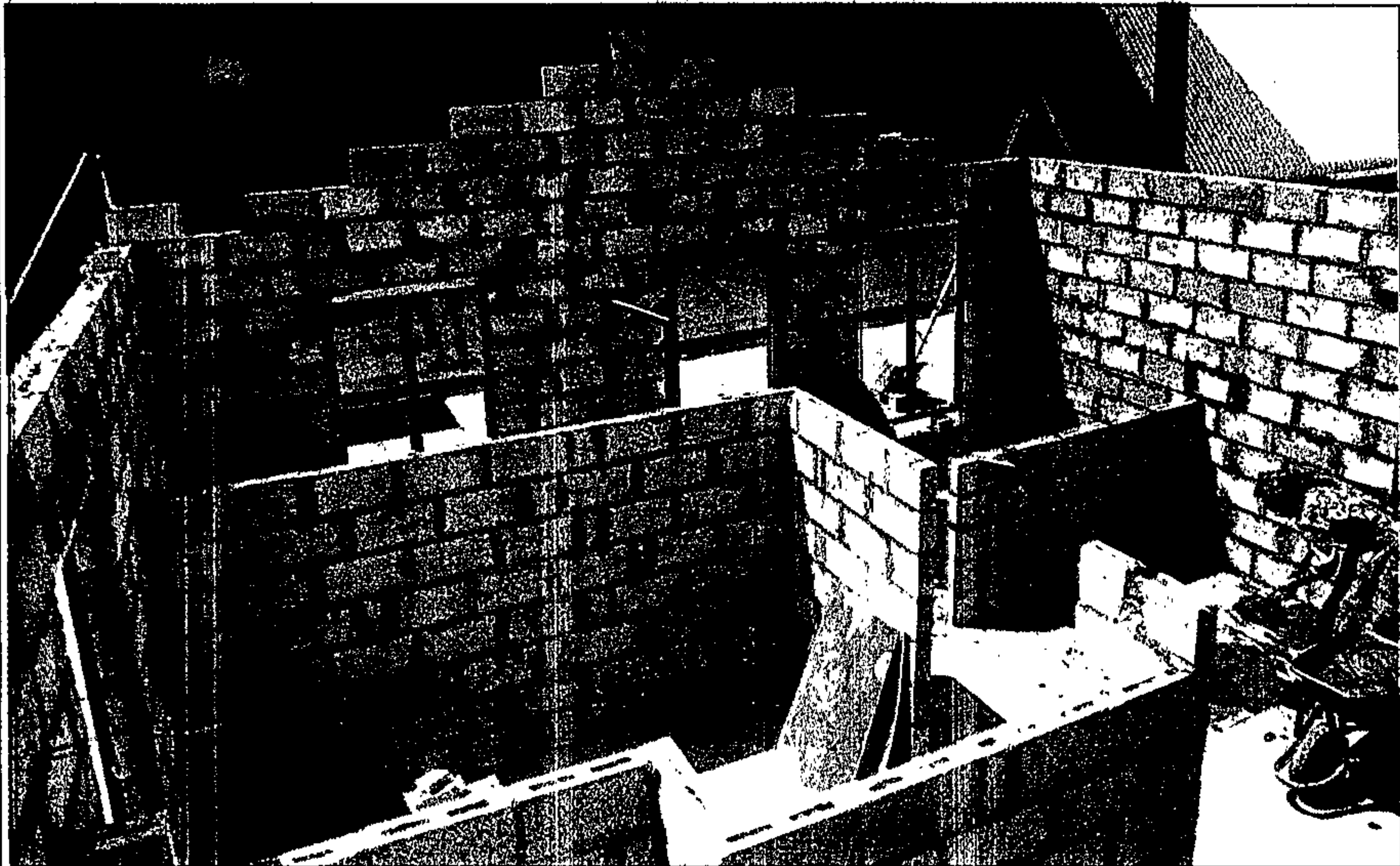
UP IT GOES . . . a peep inside an R8 000 house under construction
