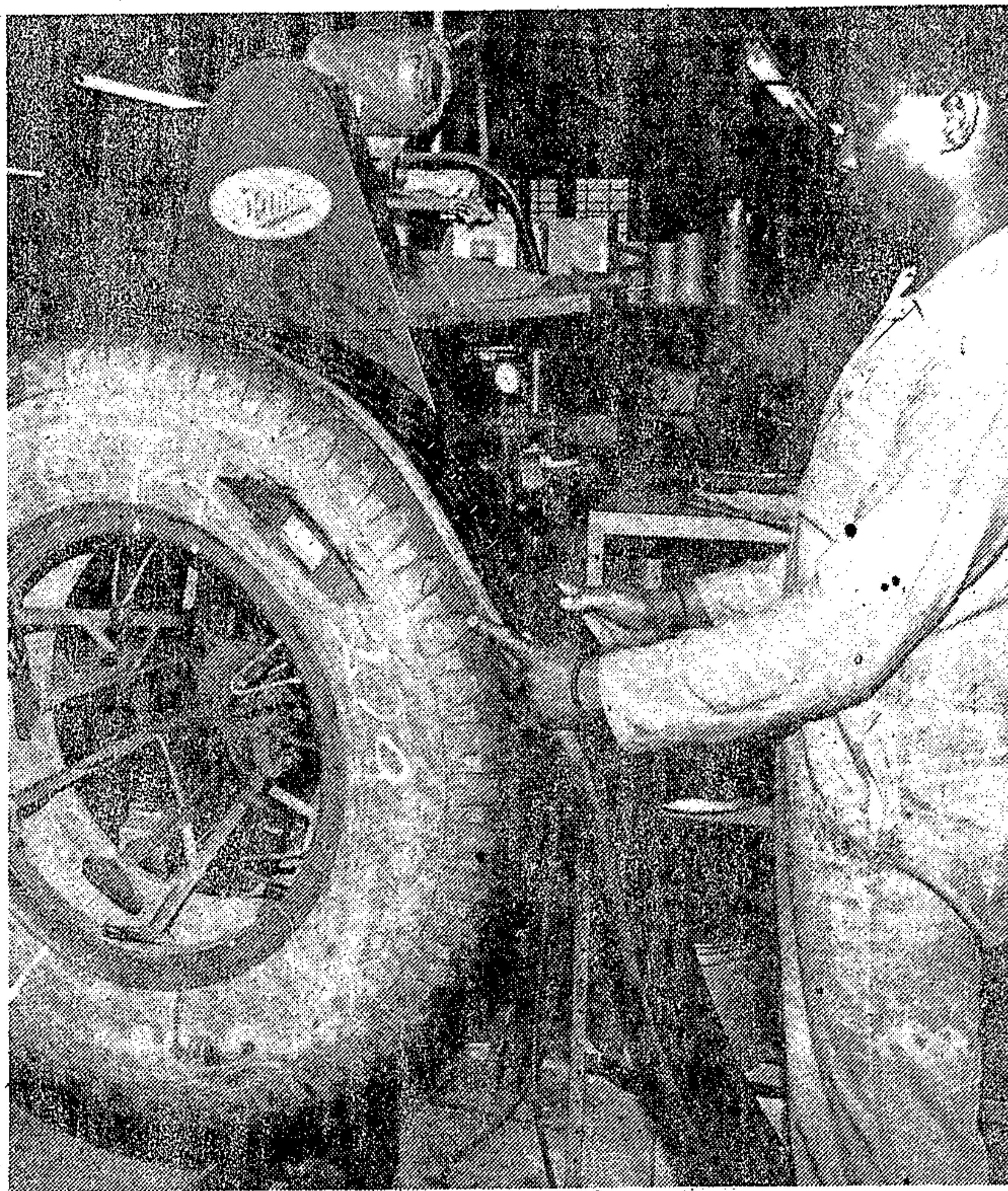
A WORKER demonstrates the simplicity of the Bandag retreading process. A pre-cured rubber strip is wrapped around the fully-inflated tyre before it is adhered by a "cold" process.
